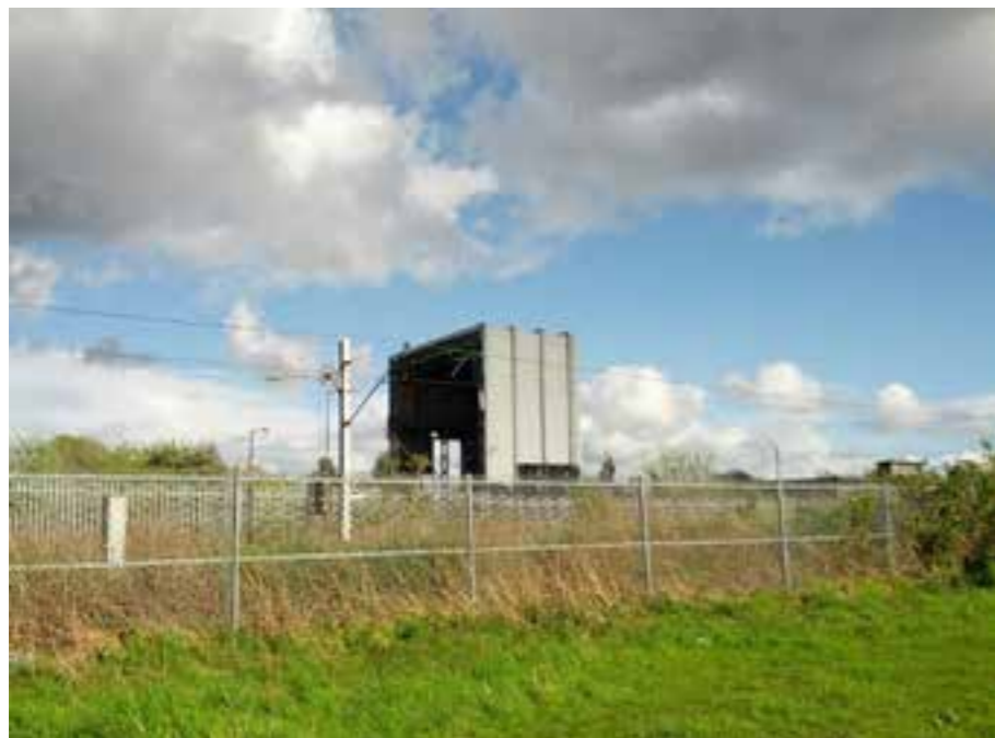
Iconic Clothier Lab testing tower prior to demoliton in 2013
